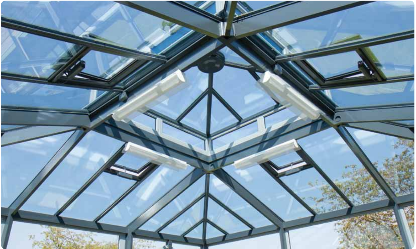
Glazed colonnade walkway, finished to a RAL specified spray-coated finish
